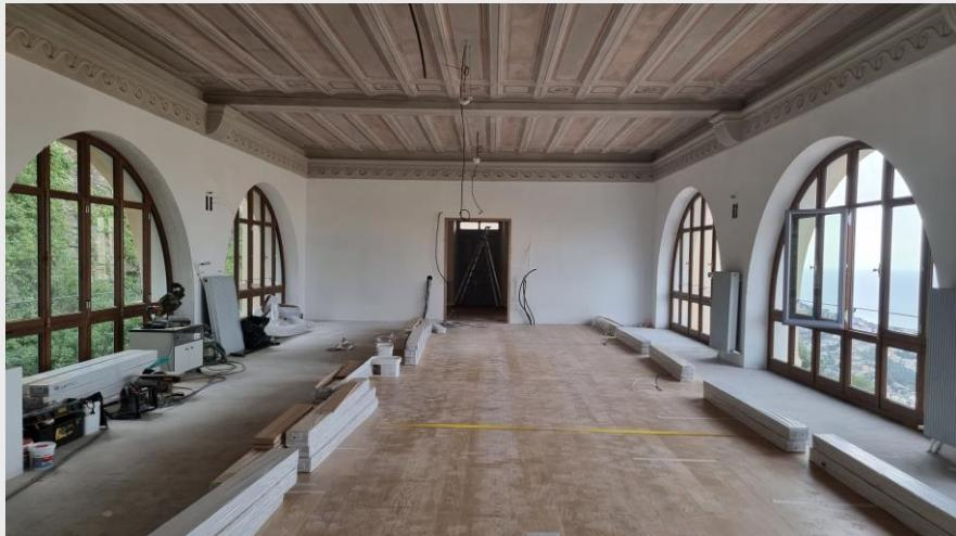
The windows are finished. The installation of the parquet floor is in progress
